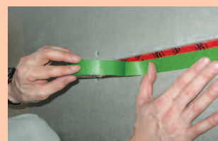
6 Installation of masking tape
