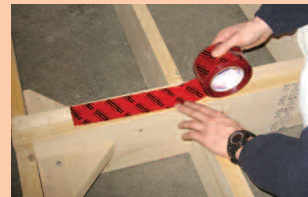
1 Installation on bond-breaking tape
