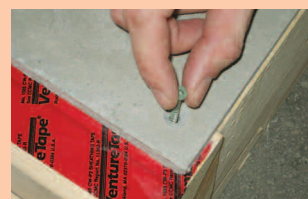
4 Hole must be larger than diameter of screw
